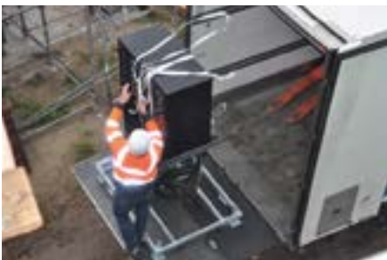
Unloading directly on the building site.
