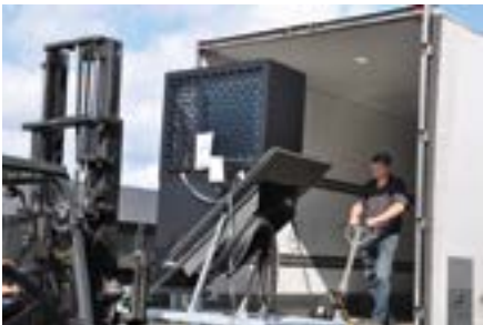
Loading the Prefab-units.
