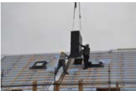
Finishing on the roof and connection indoors.
